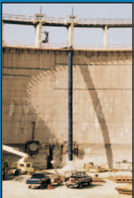
Canyon Lakes Dam, CA
